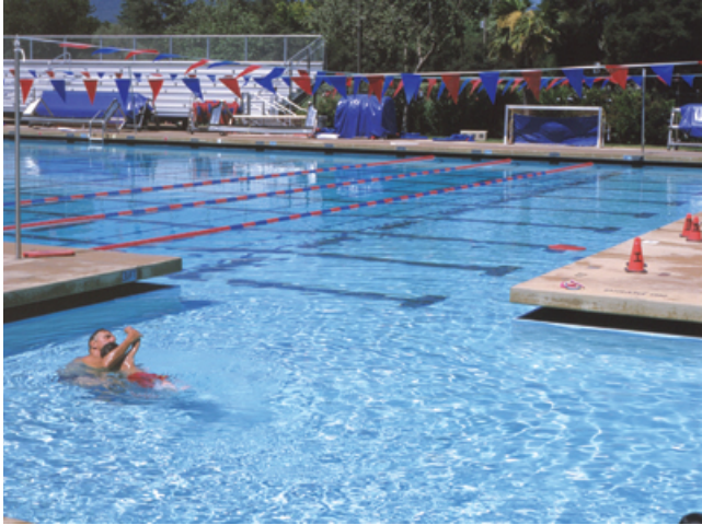
Cantilever pool deck with deep channel gutter
